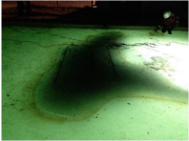
Oil trapped in cavities highlighted with underwater lights and cameras.
